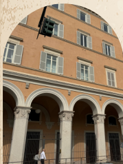
Crafted stone columns
