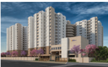
Ashraya Bengaluru - Mysore Expressway, Bidadi
