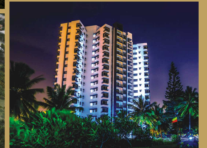
Kumar Princetown Royale - Near Jalahalli Metro Station
